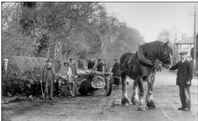
Clearing trees on Trumpington Road, c. 1930: Antony Pemberton (Stephen Brown) (stop 4).
