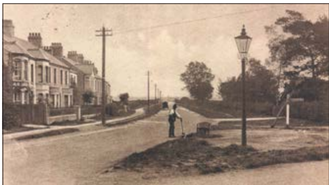
Shelford Road, Trumpington, from the junction with the High Street and Hauxton Road, c. 1914, with the first homes on the left and the cemetery on the right. Cambridgeshire Collection (stop 2).
